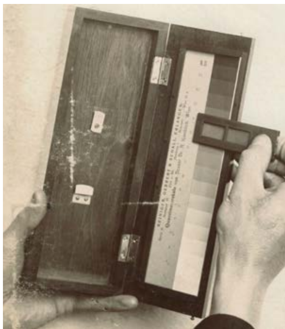
Measurement of radiation intensity (dose) using the Kienböck Quantimeter, 1905
