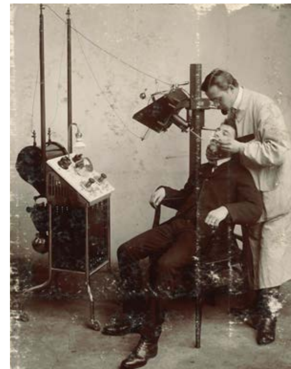
The photo of this dental X-ray system from 1909 clearly shows how close the physician and patient came to the exposed high-voltage cables
